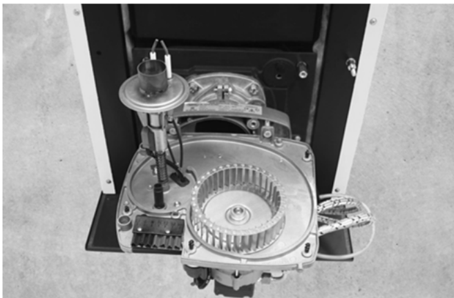
Abb. 36: Brenner in Serviceposition
